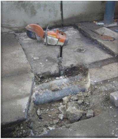
Figure 11 - Ducts in Bridge Deck
